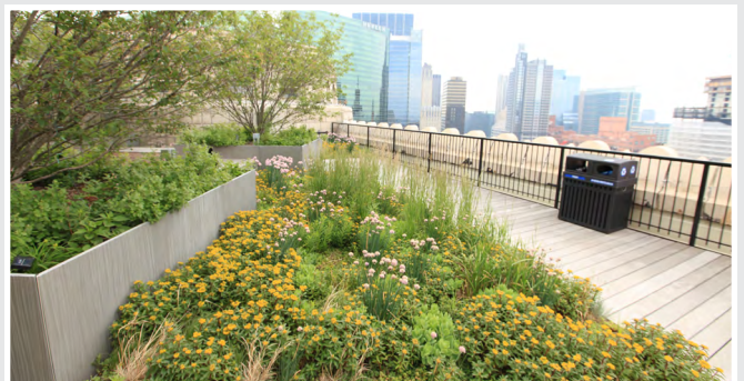
LiveRoof photo, Chicago Merchandise Mart project installed by CRCA Contractor Member, Combined Roofing.
