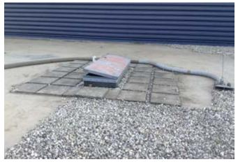
Example of access to roof via a hatch. When not in use, should be maintained in the closed position. (Photo courtesy of Safety Check, Inc.)
