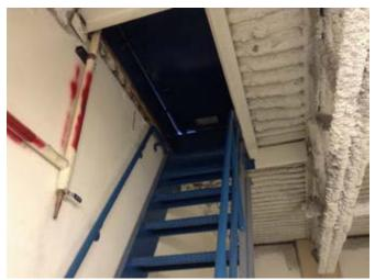
Example of the same hatch from the interior of the building with a fixed ladder. Portable ladders can also be used. (Photo courtesy of Safety Check, Inc.)
