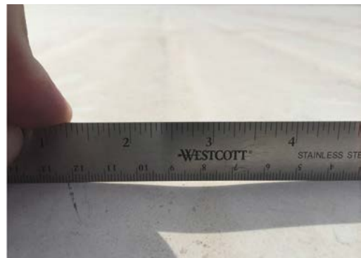
'Knit lines' in roofing, from underlying insulation. (SRI, Inc. Photos)
