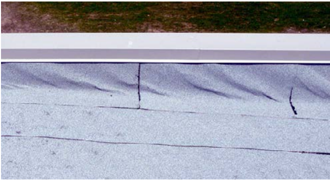
Result of shear and temperature gradient differences (Canadian Roofing Contractors Assn. Photo)
