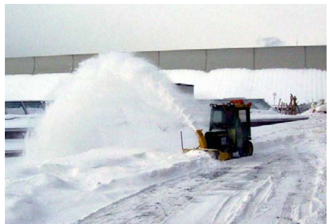
(Canadian Roofing Contractors Assn. Photo)
