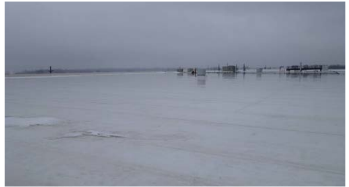
White Roof (SRI, Inc. Photo)
