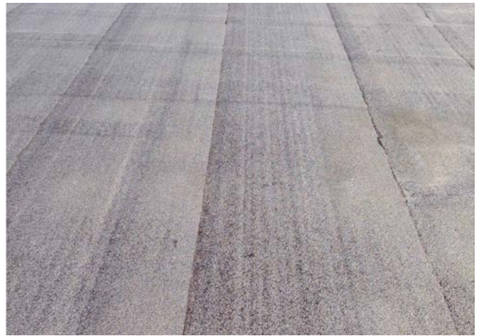
“Laning” of granules on modified bitumen roof covering. (SRI, Inc. Photo)
