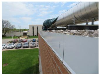
Photo 1: Edge metal must be higher than ballast (2-inch minimum). (Raths Raths & Johnson photo)
