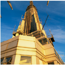
Empire State Building, New York, NY
