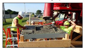
Photo 1. A large general contractor was utilized to provide concrete slab assembly, placement and finishing. These slabs are the exterior slabs, exposed to the full weather at SRI Consultants facility
