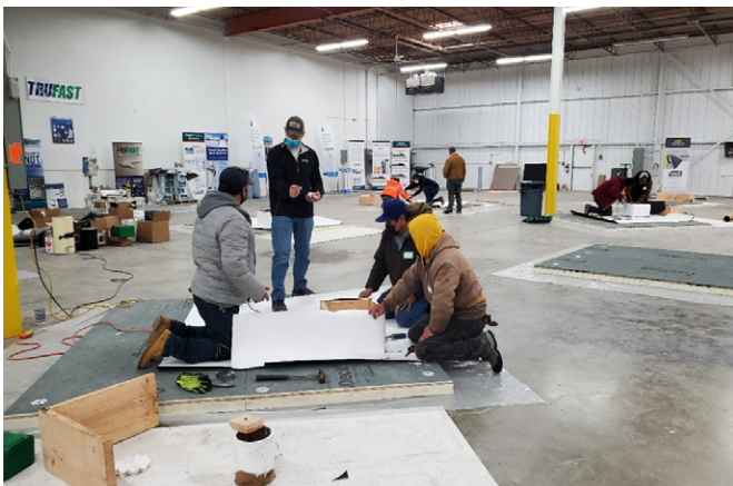
Comstruct Sales LLC photo
